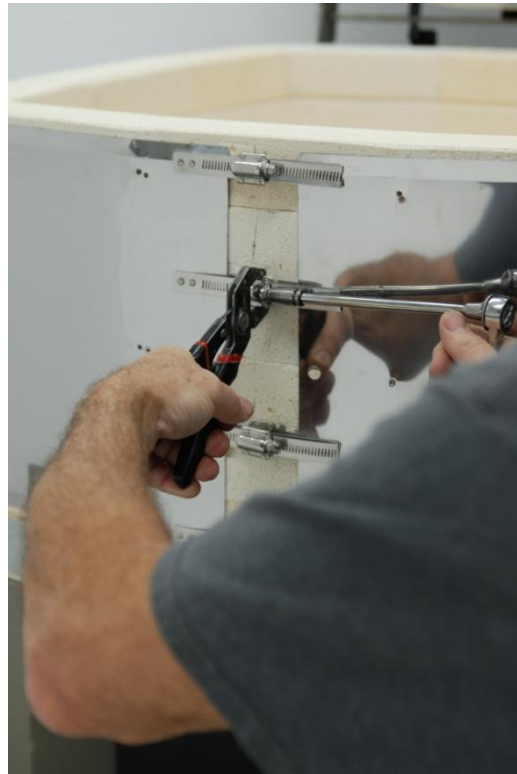
Figure 6 – Tightening with 5/16” Socket
